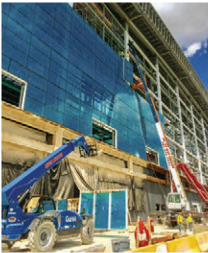
'The Pearl of Miami' Norwegian Cruise Line Terminal B north façade.
