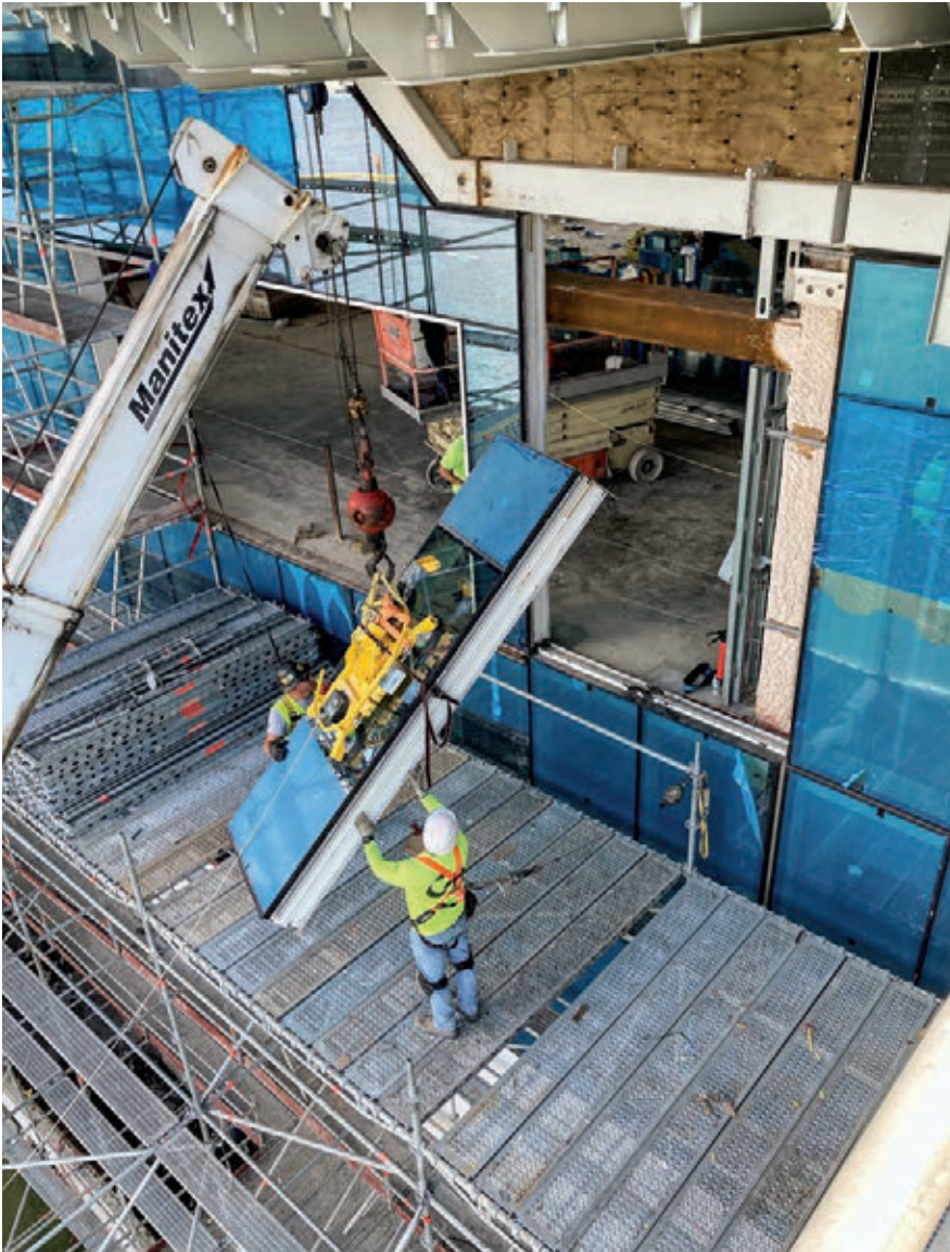
Port of Miami Virgin Cruises Terminal V frames installation.
