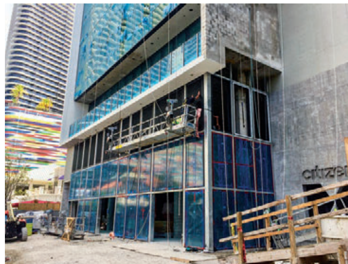
CitizenM Brickell installation.
