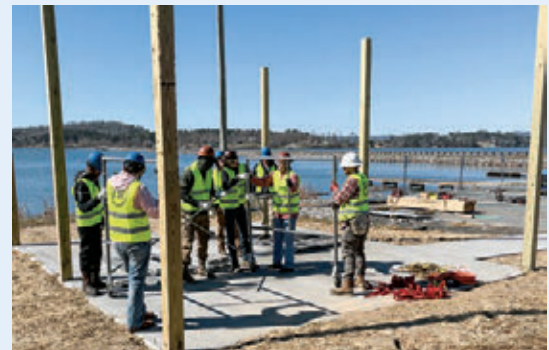
The skills of the ironworker apprentices learned while building the pavilion fit perfectly into their training schedule.
