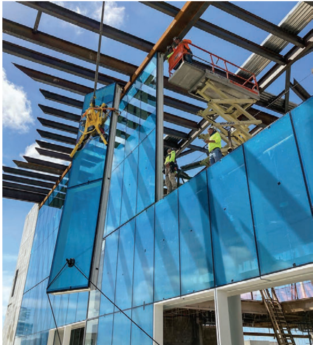
Port of Miami Virgin Cruises Terminal V frames installation.
